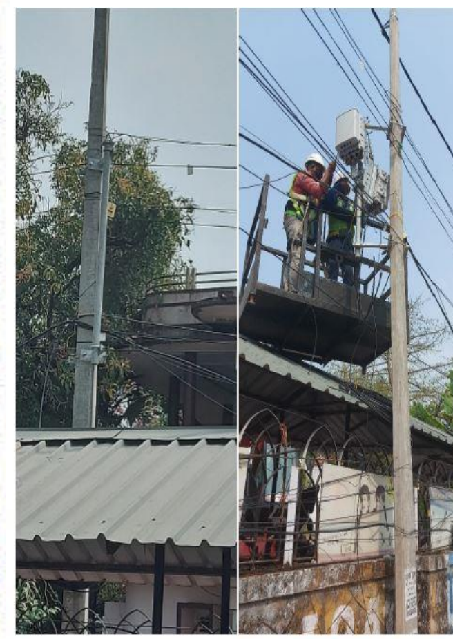
Small Cell Power tapping on Electric Poles by KSEB
